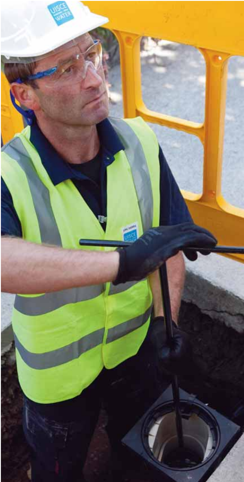
■ First Water meters being installed by Irish Water employee in Maynooth.
